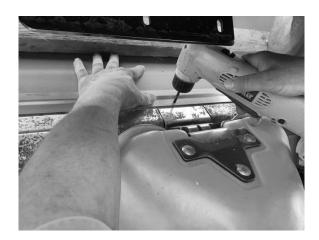
Install the 3/16" rivets by drilling 13/64" hole and installing one rivet at a time. Pay careful attention to hold down location as you work your way from one end to the other to keep
