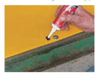
Use the silicone sealant supplied to seal around each bolt head and to fill in any unused holes.
